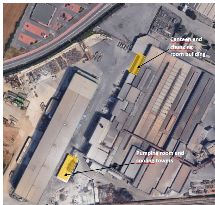
Figure 2 - the productive plant and the place of pumping room and canteen and changing room building, the distance is about 130 m.
