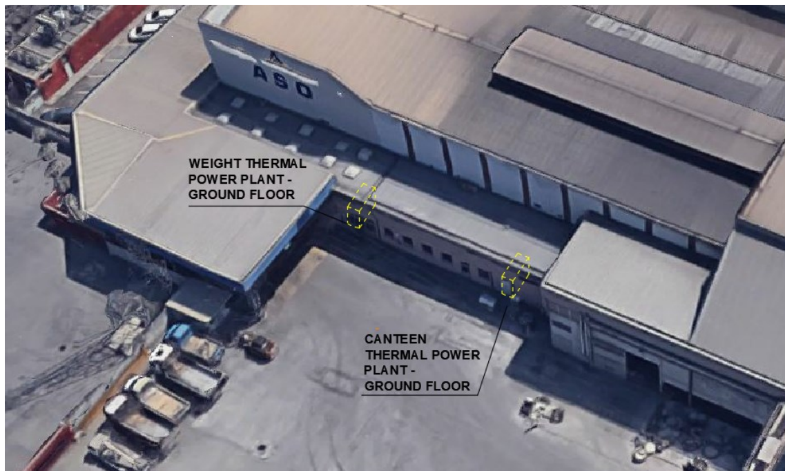
Figure 3 - location of the former ASO thermal plants
