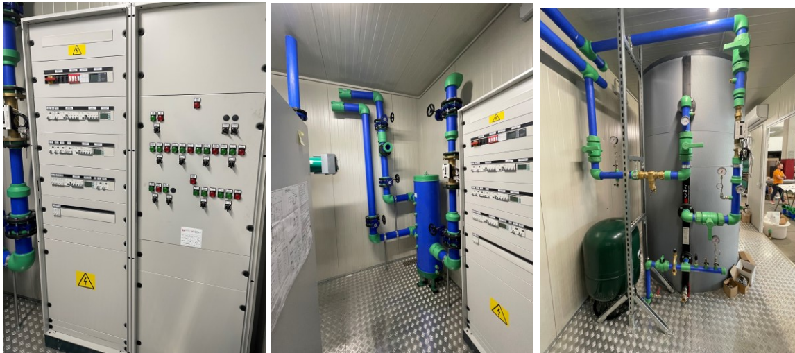
Figure 22: construction works (switchboards, hydraulic separator, stratified tank).
