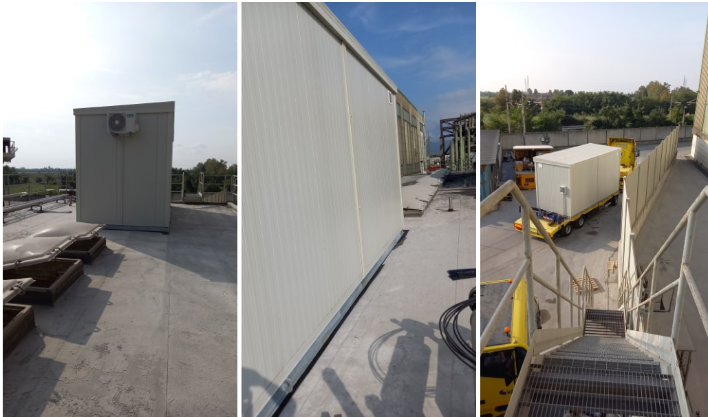
Figure 18: construction works. Delivery of the containerized hydraulic kit.
