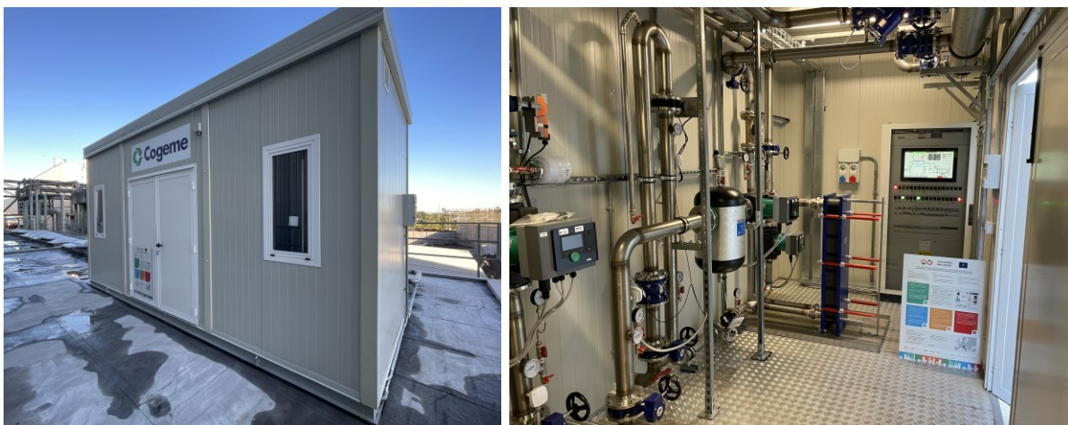
Figure 20: construction works (hydraulic kit).
