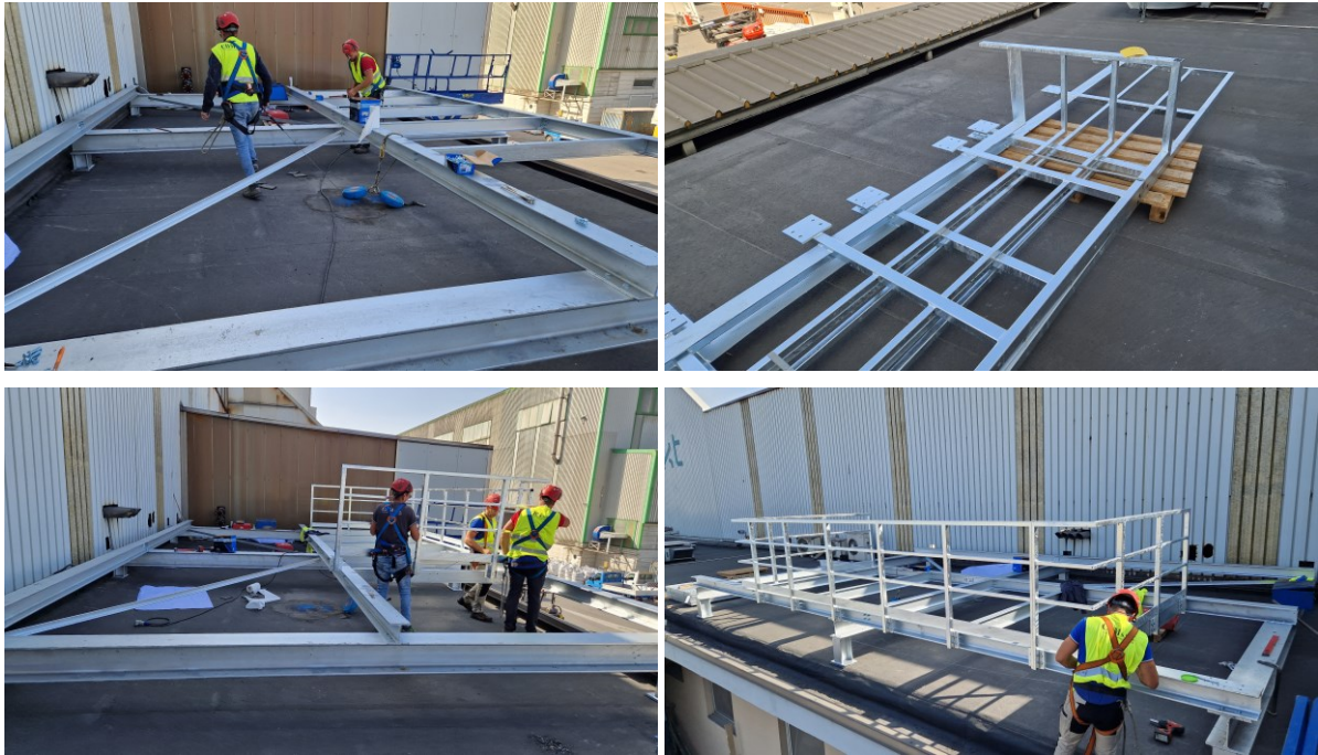
Figure 13 construction works for the steel structure sustaining the heat pump container.
