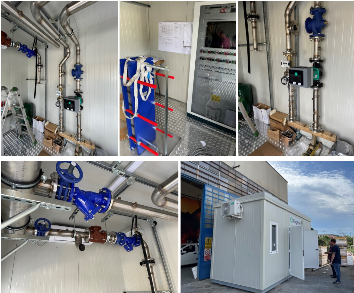
Figure 19: construction works (hydraulic kit).
