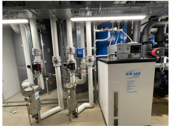
Die Installation in Heerlen
